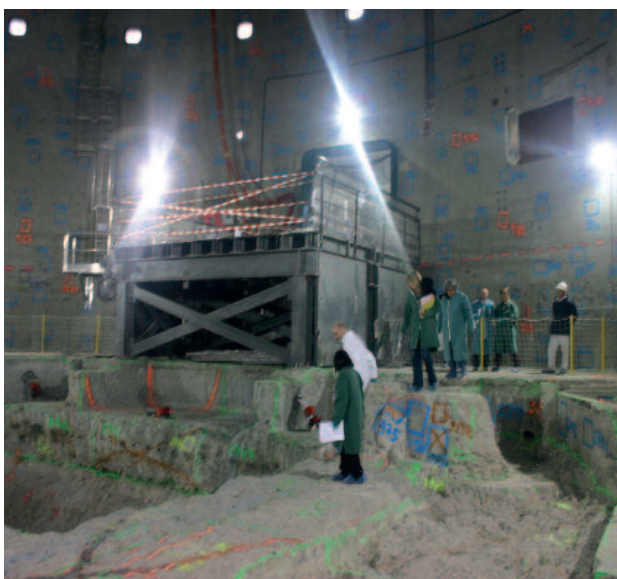
ASN inspection of the delicensing of the SILOE reactor basemat – December 2011
