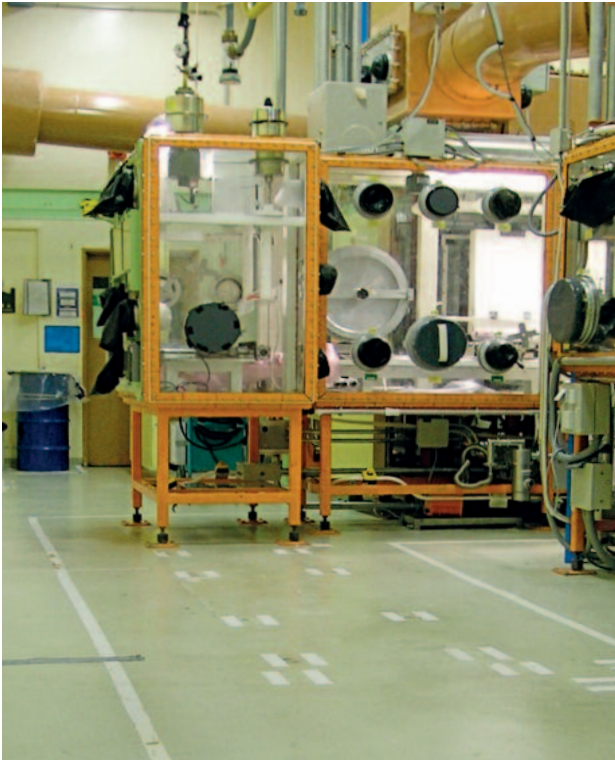
The enriched uranium processing facilities (ATUEs)
