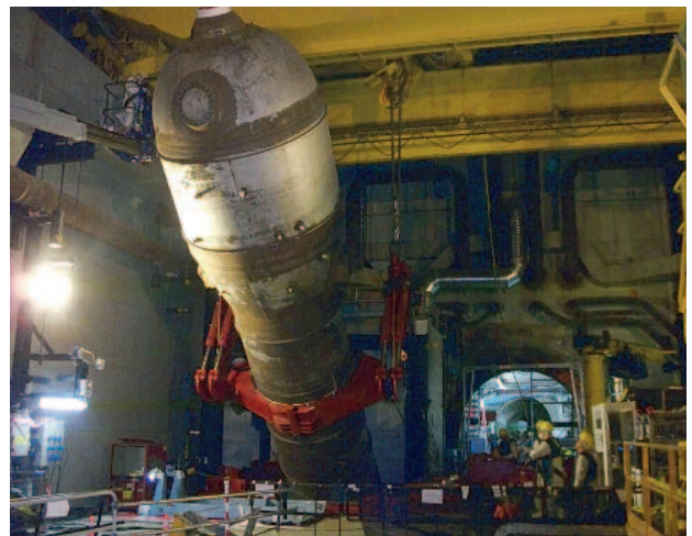
Removal of a steam generator at Chooz – October 2011
