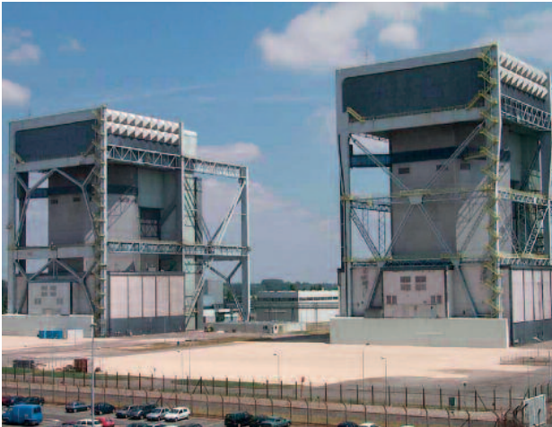
Views of the Saint-Laurent-des-Eaux NPP before and after the works
