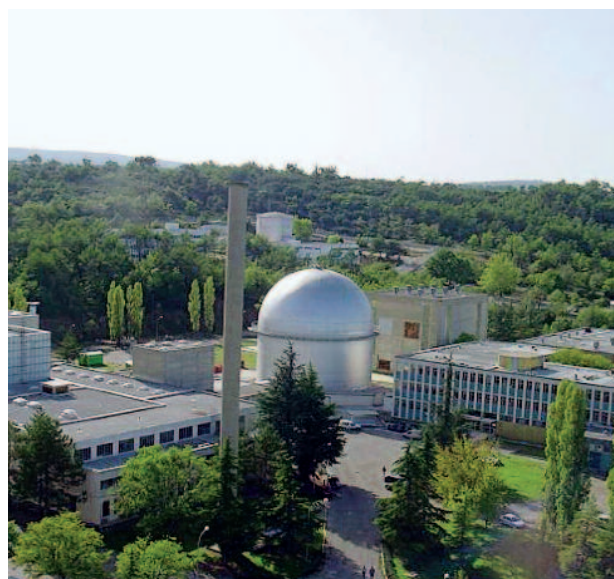
View of the RAPSODIE reactor
